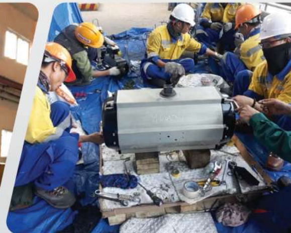
ACTUATOR VALVE MAINTENANCE
