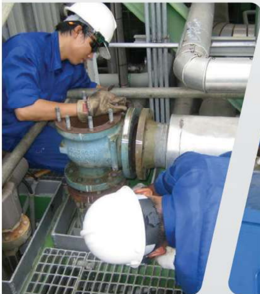
SAFETY VALVE MAINTENANCE
