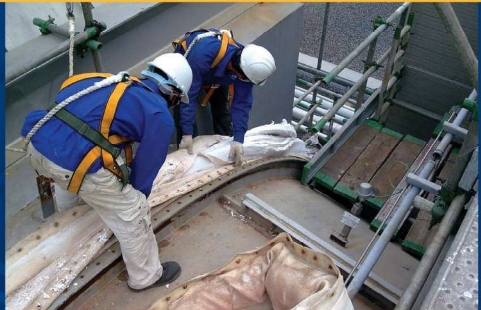
EXPANSION JOINT REPLACEMENT
