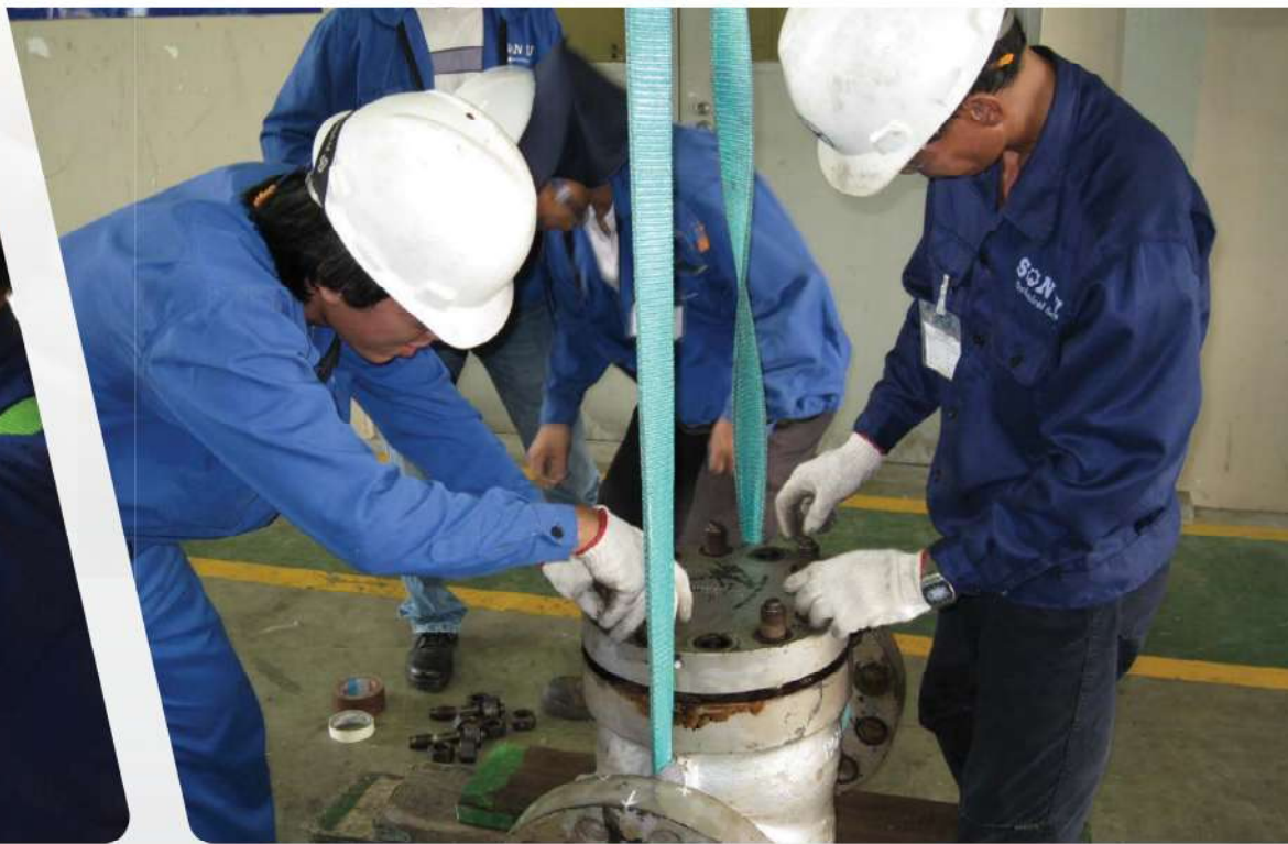
MINIMUM FLOW VALVE MAINTENANCE
